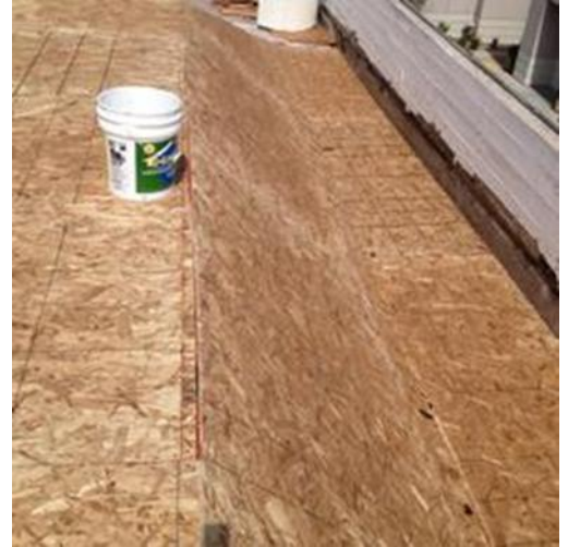
New sheathing installed
