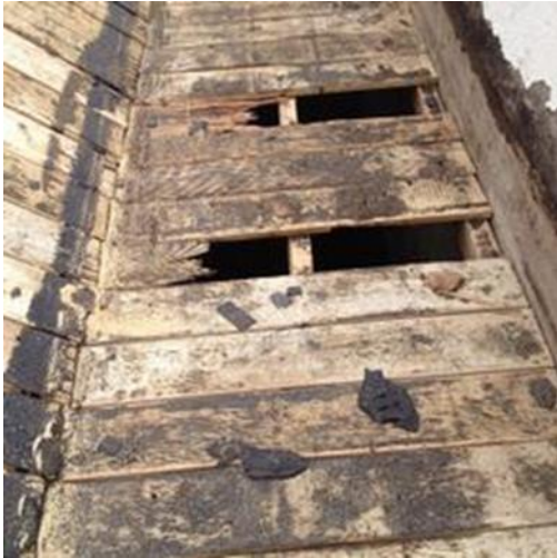
Roof condition prior to repair
