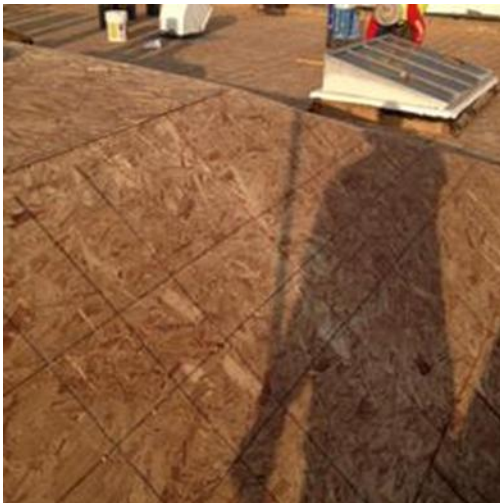
Another look at the new sheathing
